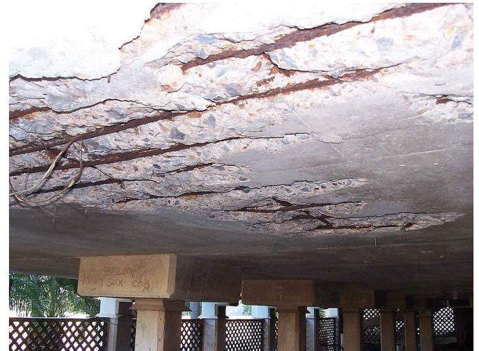
Figure 2: Showing what happens if cover is not adequate
