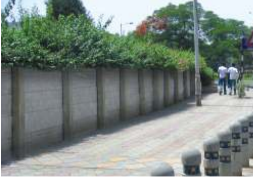
Six Feet Boundary Wall
