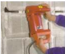
Cement Blocks... No Problem
