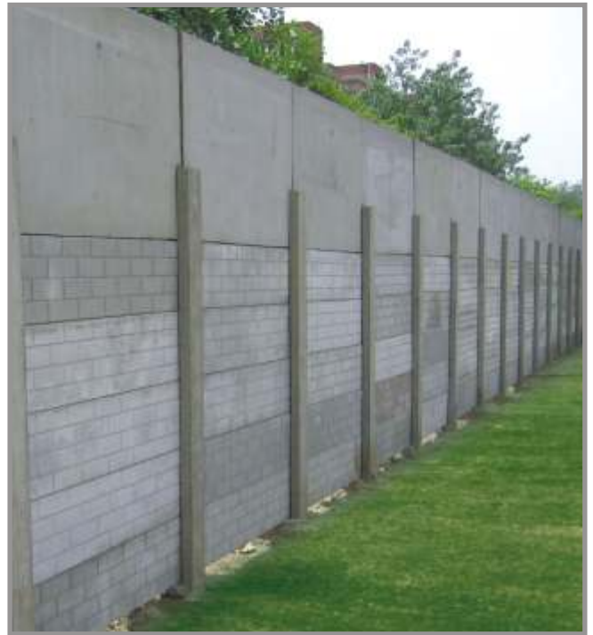
Eight Feet Boundary Wall
