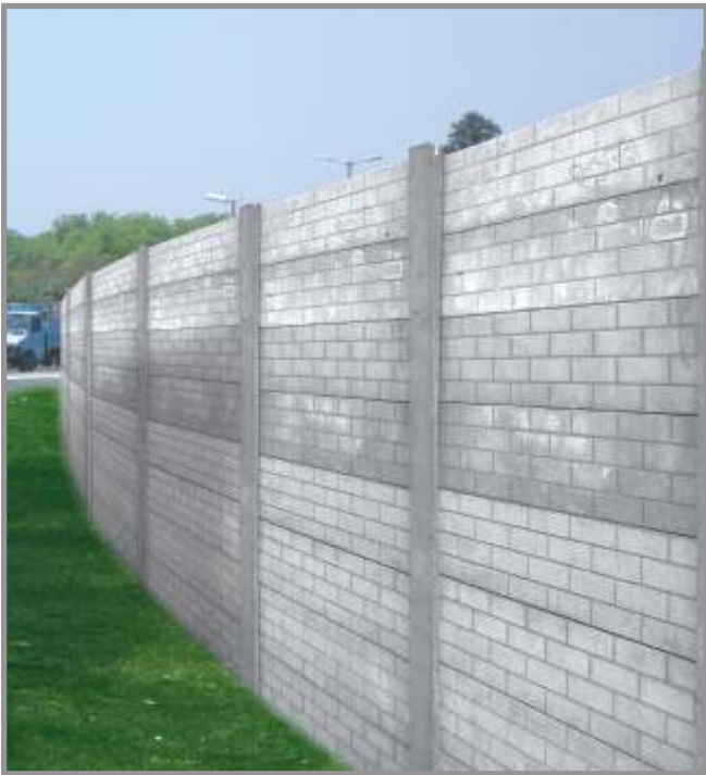
Eight Feet Boundary Wall
