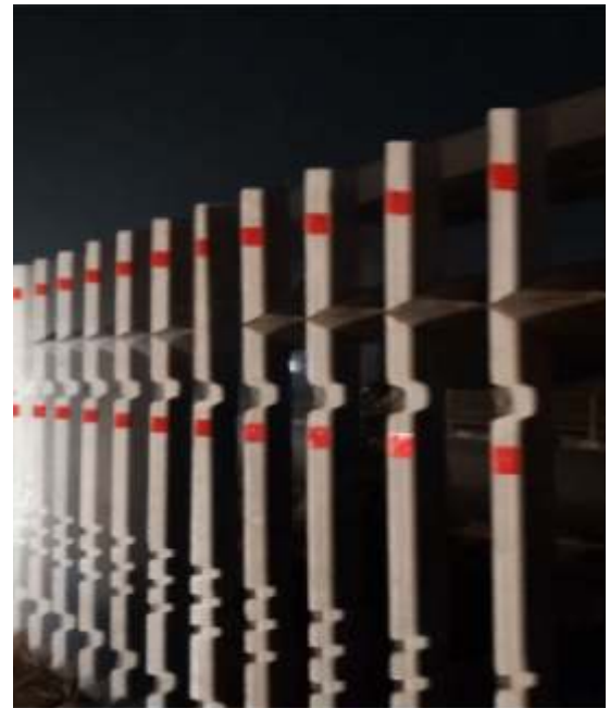
“Reflective Tape can be affixed to this fence for night time visibility
